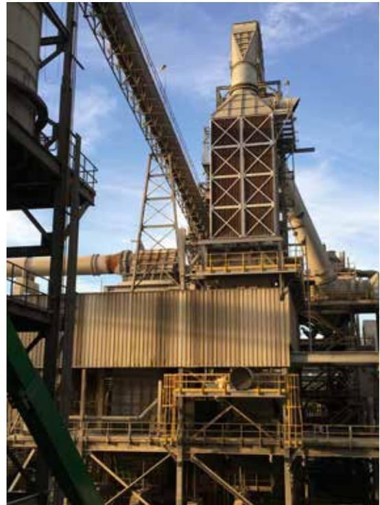
Once the module is isolated from the process stream, the Scheuch Impuls (pulse jet) bag cleaning utilizes low-pressure compressed air, that passes through engineered nozzles and venturis, entraining more ambient air than more traditional pulse jet arrangements. The tuned nozzles ensure that each bag in the row receives the same volume of cleaning air, ensuring even, effective bag cleaning and consistent emissions and pressure drop performance over the life of the bags.
